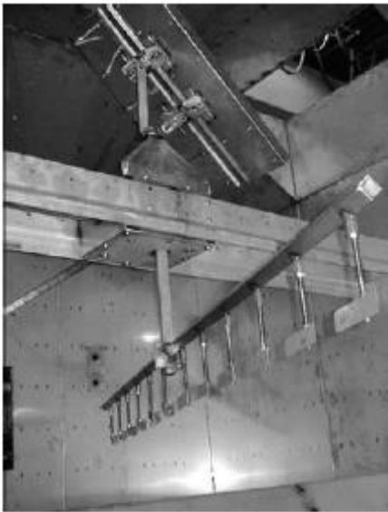
Figure 12-2. Counterflow cooler with rotating arm.
